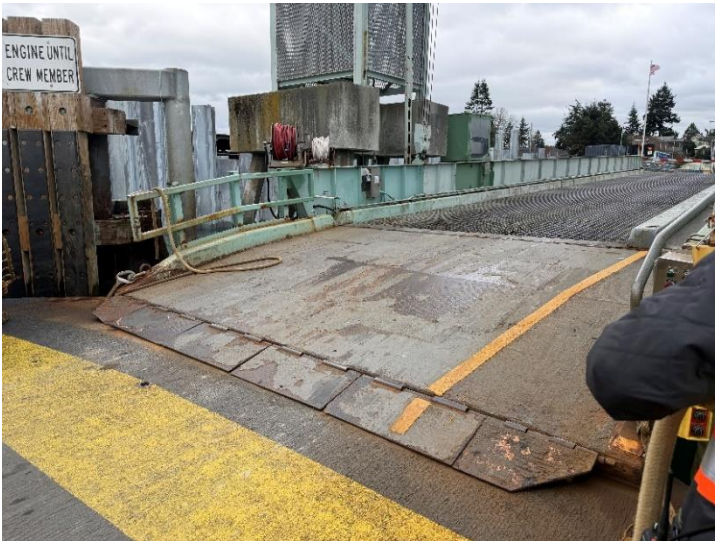
Anacortes Bridge Apron
